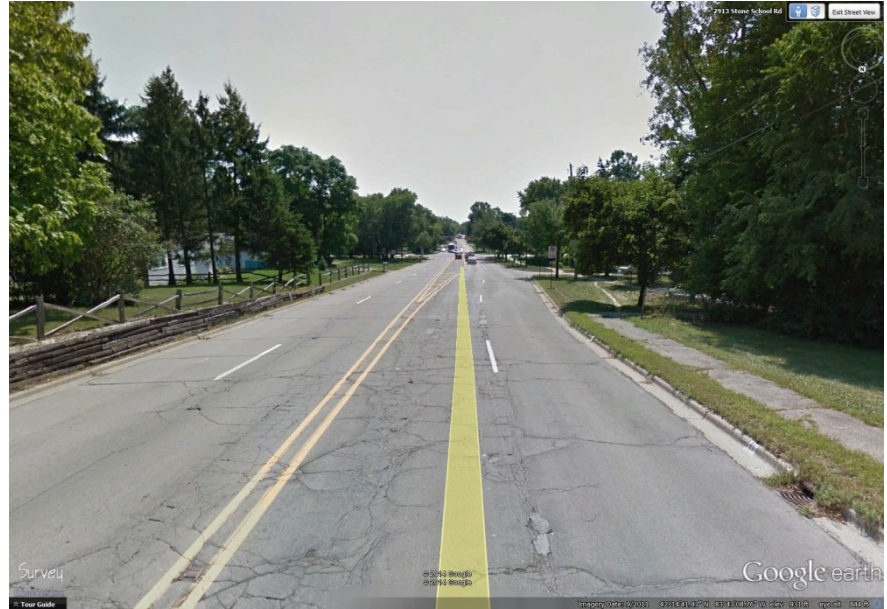
Site #1, South on Stone School Road
