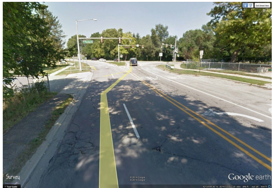
Site #1, North on Stone School Road towards Packard
