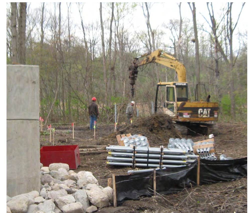
Rip Rap and Silt Fence In Place Prior to Construction - Photo Credit: CDF
