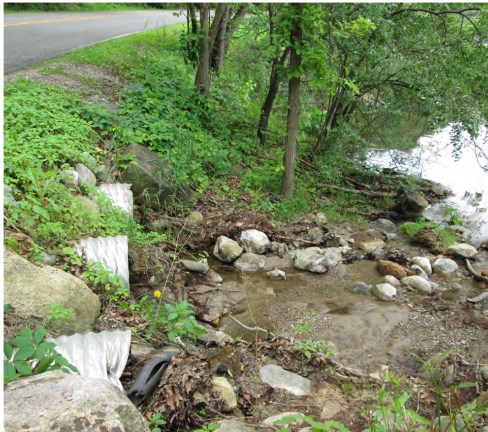
Heavy sediment build-up along Huron River Drive - Photo Credit: CDF
