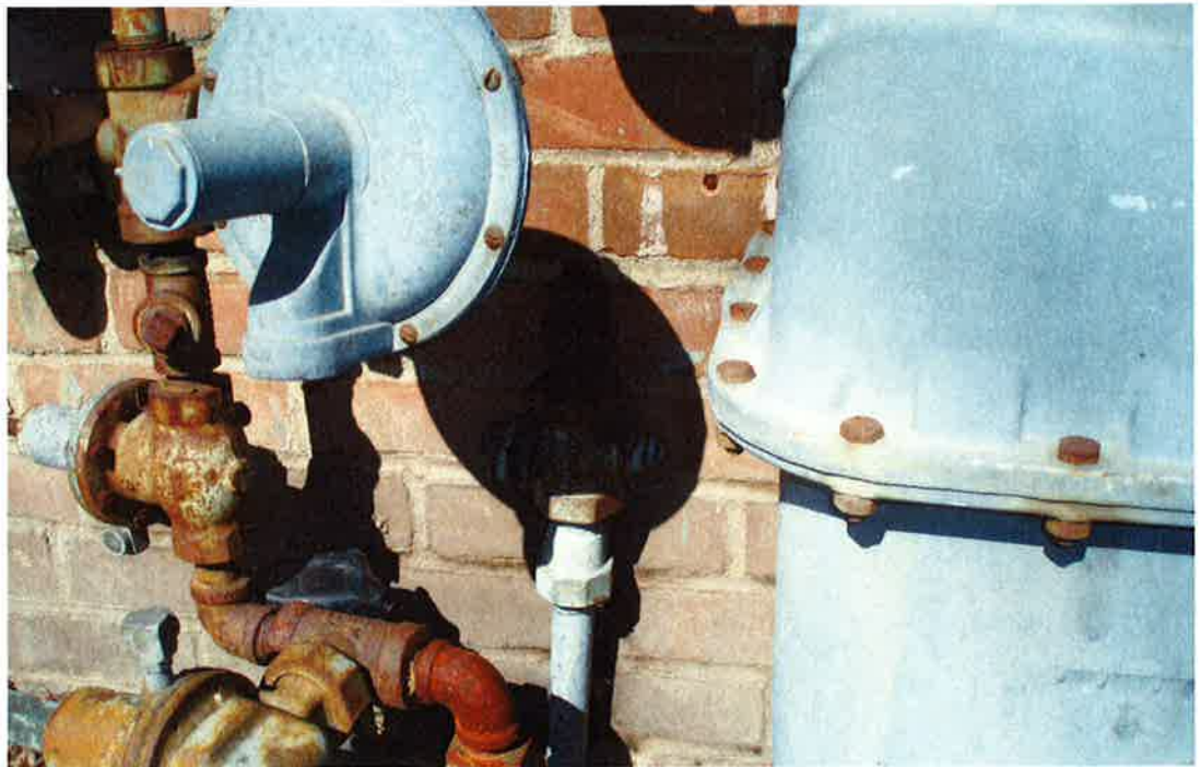
A GENERAL VIEW OF THE VENT PIPE
