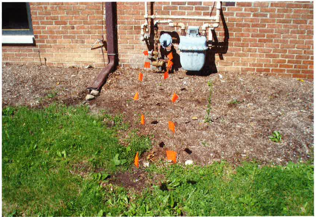
A GENERAL VIEW OF THE APPROXIMATE UST PIPING LOCATION
