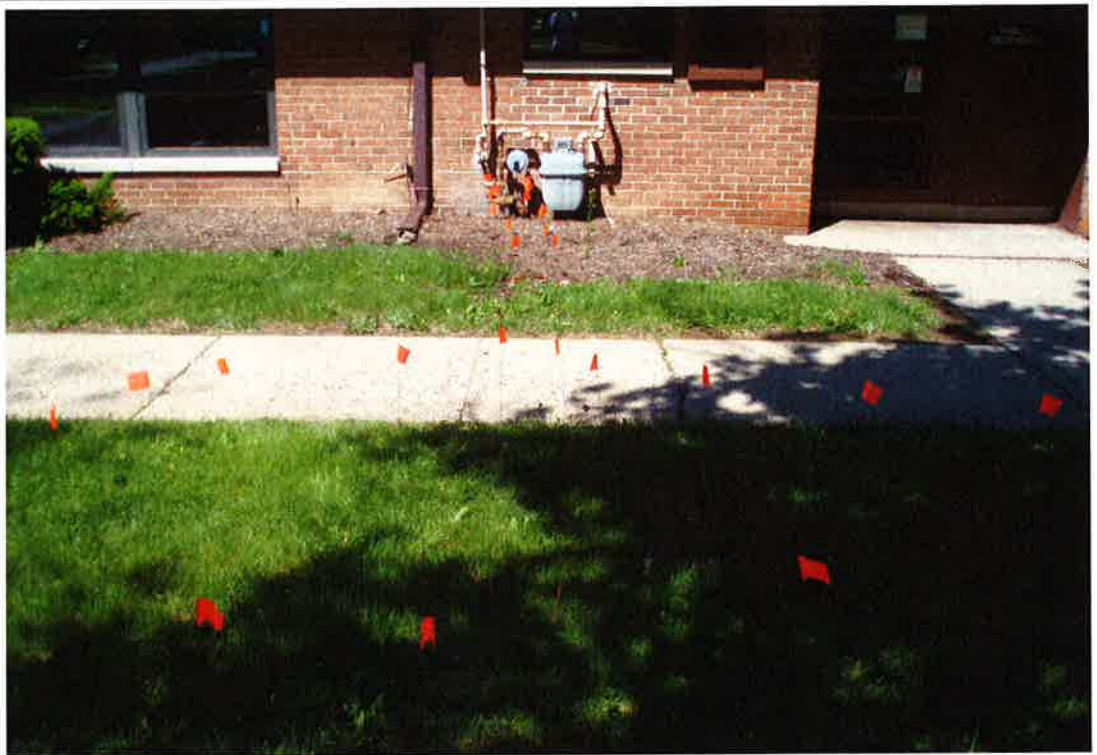
A GENERAL VIEW OF THE APPROXIMATE UST LOCATION
